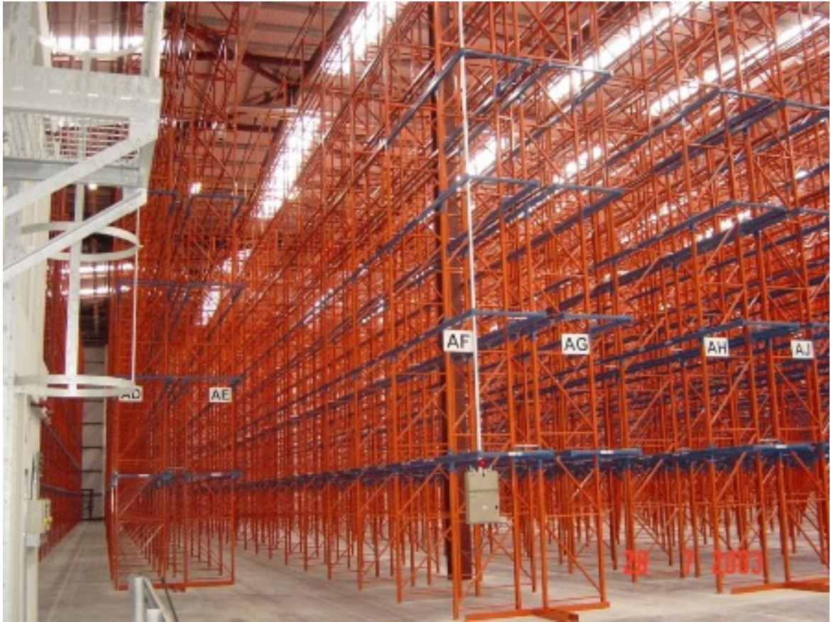
Figure 6 – VNA Racking (empty)
